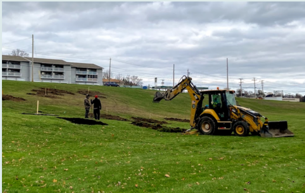
Westcott Reservoir Pit Excavation
