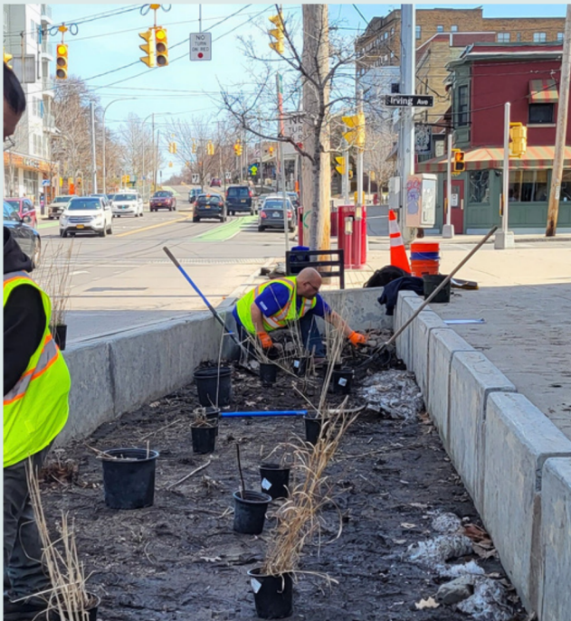
Brent working in a rain garden on East Genesee Street.
