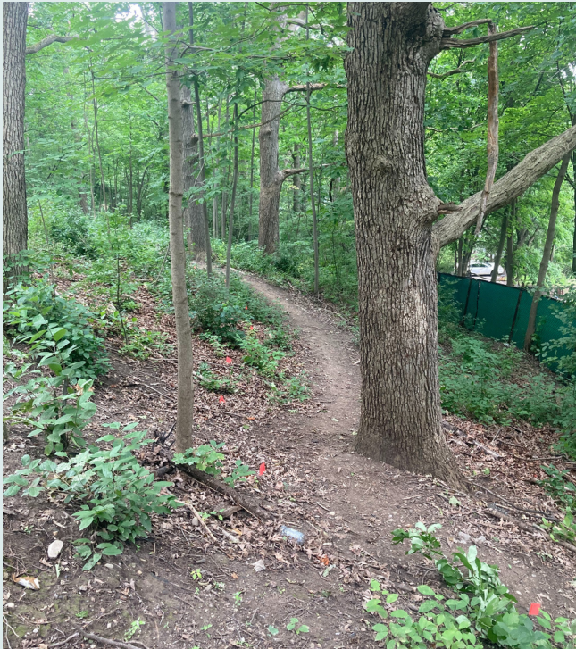
OEC crews create a sustainable trail by building a half bench trail tread. This helps prevent further erosion and promotes better runoff for water along the slope. Before- Left, After- Right.
