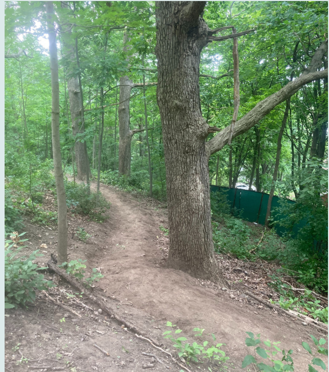
OEC crews create a sustainable trail by building a half bench trail tread. This helps prevent further erosion and promotes better runoff for water along the slope. Before- Left, After- Right.
